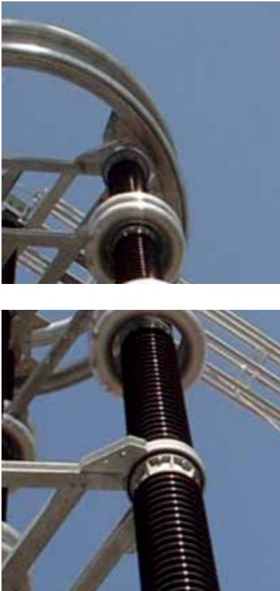
In IEC60815 the basic pollution levels are defined qualitatively with examples of typical environmental situations. The corresponding minimum nominal creepage distance is given in mm/kV.
